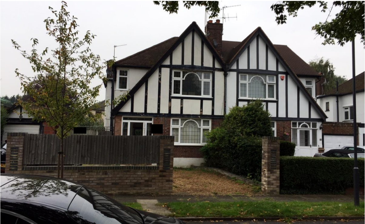
Front elevation of application site and the adjoining property No. 15 Sherington Avenue.
